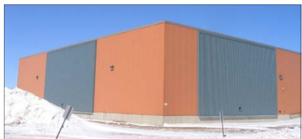
Solar cladding installed on the southeast and southwest wall of Building 60.
