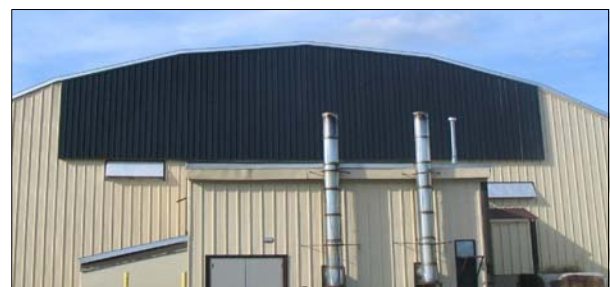
Rocky Grey SolarWall panels were chosen for the hangar buildings to match an existing color
