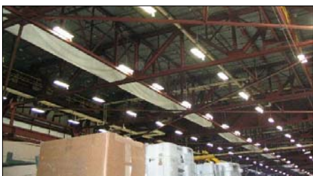
In buildings with heat stratification at the ceiling, the SolarWall system was connected to wall mounted fans and perforated distribution ducting to disperse the hot air at the ceiling around the building.
