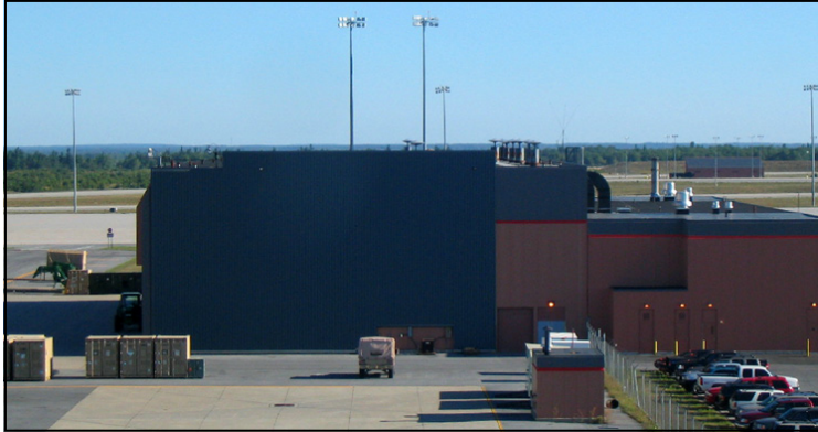
Left, the completed SolarWall system at Fort Drum's building 2074, and above building 1750
