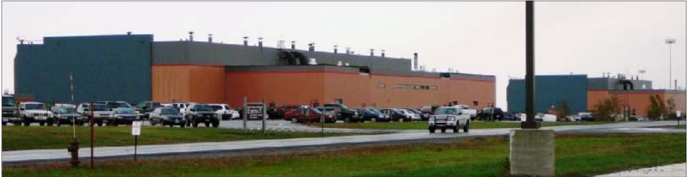
The world's largest collection of solar air heated buildings is located at Fort Drum, New York
