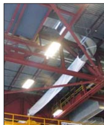
In buildings with heat stratification at the ceiling, the SolarWall system was connected to wall mounted fans and perforated distribution ducting to disperse the hot air at the ceiling around the building.
