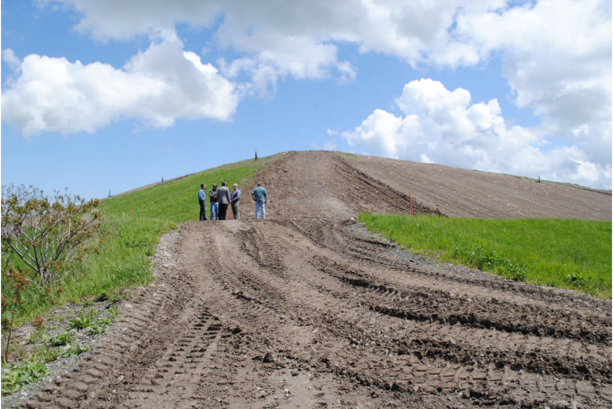
Eleven solar panels will be place on the southern facing slope, shown above, of the closed west side landfill at the Buyea Rd Landfill site in the Town of Lincoln.
